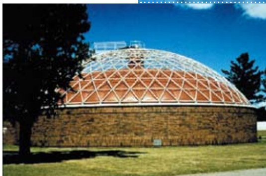
The Dystor Bio-Gas Holder can hold up to three times more gas than alternatives.
